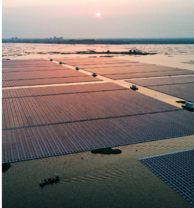
A solar farm floats on a lake that formed after the collapse of a deep coal mine in Huainan, China.
