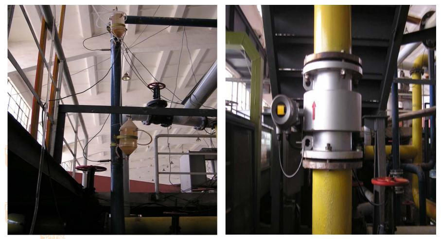
the isolation pot and differential pressure The electromagnetic flow meter for the sensor discharge and the flow velocity test
